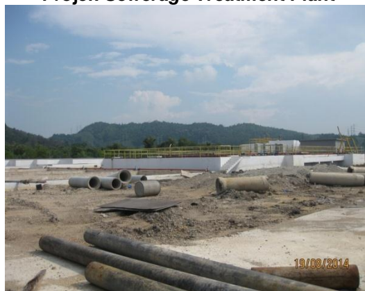
Gambar 2.2 Projek Sewerage Treatment Plant
